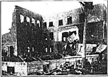
View of a modern macaroni plant after fire had completed its destruction.
